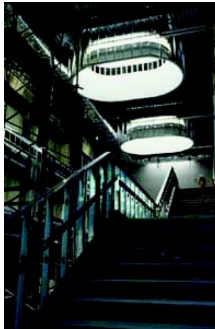
Duffield Hall's atrium under construction
